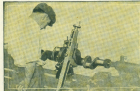
Fig. 58. Truing Crankshaft Throw Bearings with a Weber Tool Attachment.
