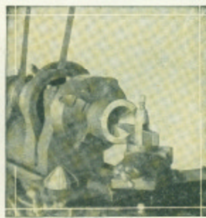
Fig. 65. Boring the Taper of a Conical Die.
