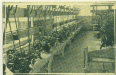
Fig. 5. A Practical Method of Installation for Bench Lathes in a Modern Shop.
