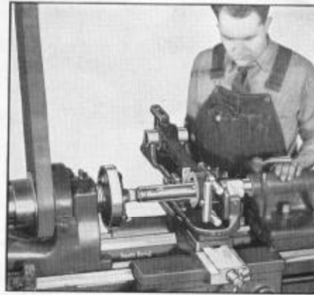
Fig. 38. Boring a connecting rod.
